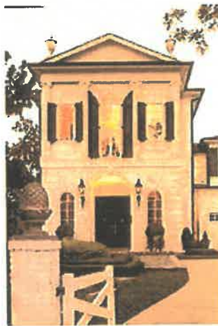
Small carriage house on possible larger property.
